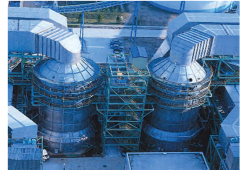
▲ The desulfurization unit is auxiliary facilities of thermal power plants designed to prevent air pollution. In the flue gas desulfurization unit at coal fired power generation plants, chlorine in the fuel condenses to create a corrosive environment of high concentration chloride. In environments where the chlorine ion concentration exceeds 10,000 ppm, the super stainless steels 254NM and 74N, and highly corrosion-resistant Ni alloys NW276 and NW22 are used to reduce the cost and to extend the service life of the unit.
