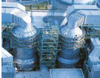
Flue gas desulfurization equipment at a coal fired power plant
