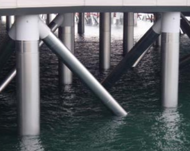
The sheath material of the bridge pier for runway D at Haneda Airport
