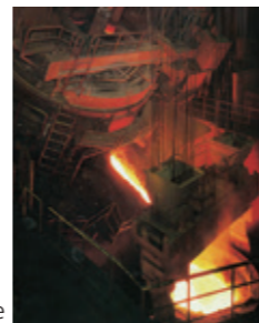
Previous electric arc furnace
