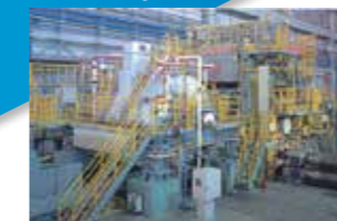
New hot rolling mill
