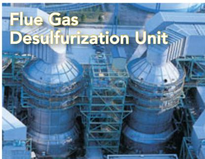
The flue gas desulfurization (FGD) unit is part of the auxiliary facilities of thermal-power plants designed to prevent atmospheric pollution.
