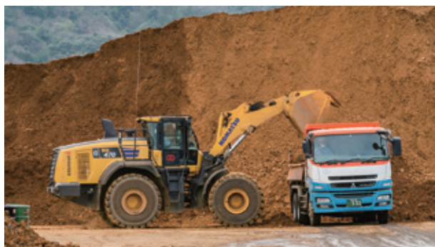
Oheyama Plant An ore yard
