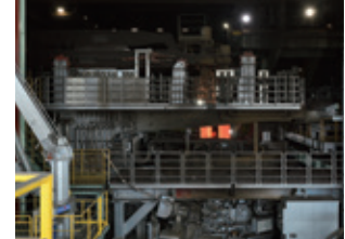
New electric arc furnace ("E furnace")
