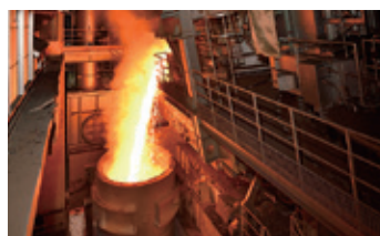
New electric arc furnace ("E furnace")
